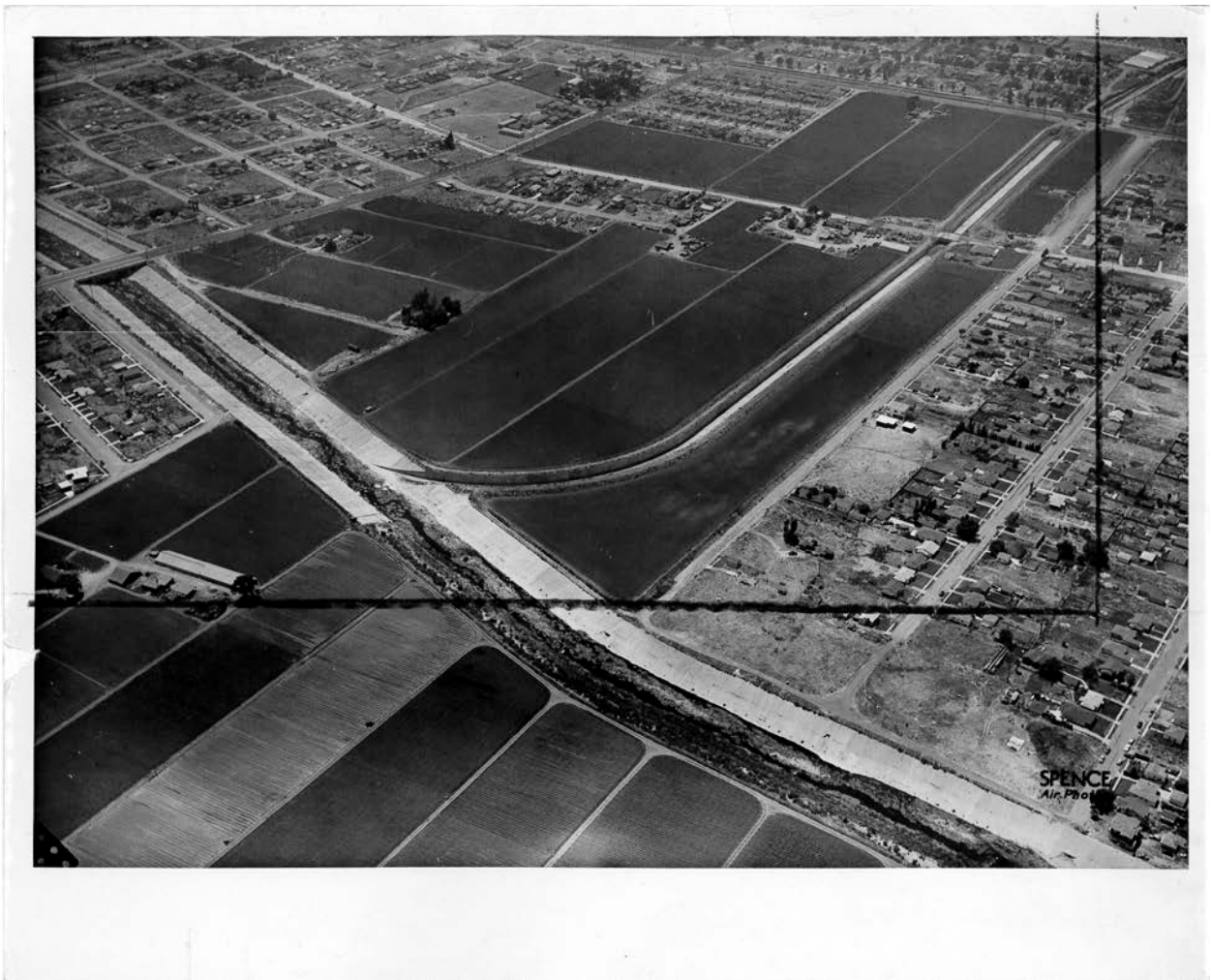
Figure 1: Aerial view of Mar Vista Gardens Site prior to construction. Undated. Courtesy of HACLA.
